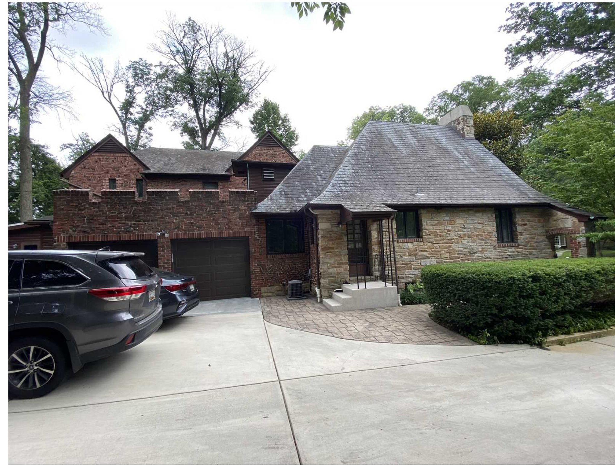
VIEW FROM THE WEST
